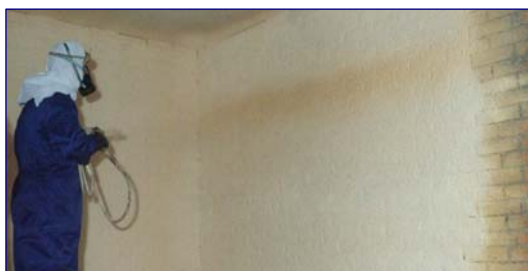
Picture 23: Spraying over a masonry wall
